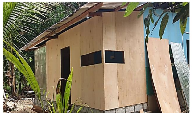
Jose mama's house being rebuilt
